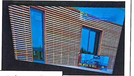
Horizontal wood slat exterior cover
